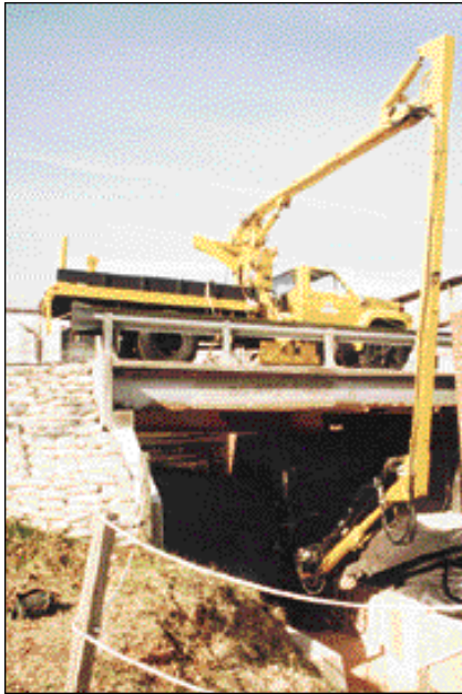
The truck-mounted Robotic Bridge Maintenance System is field tested.
