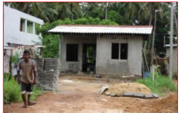
new housing construction in Sri Lanka
