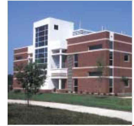
NC State's Toxicology Building on Centennial Campus
