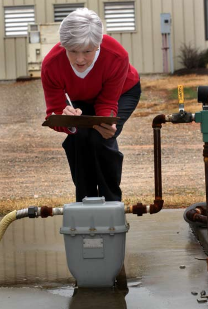
Dr. Jeanne Koger records meter readings as a nearby furnace converts hog waste into ash for fertilizers and gases to power the furnace. ●
