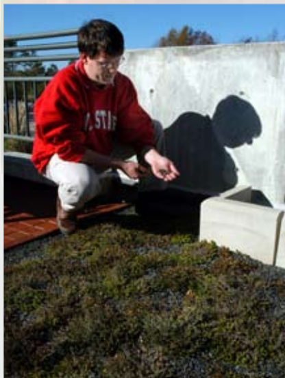
Dr. Bill Hunt works with developers on designs that limit stormwater runoff, such as this roof garden atop a building at NC State’s J.C. Raulston Arboretum. ●
