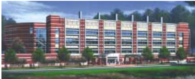
New building on Centennial Campus for Chemical Engineering and Materials Science Departments •
