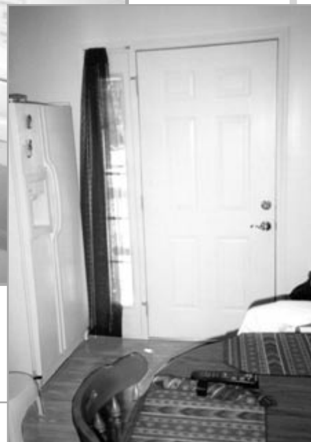
Sidelight next to entry door allows full view of visitors from any height whether tall or short or standing or seated.
