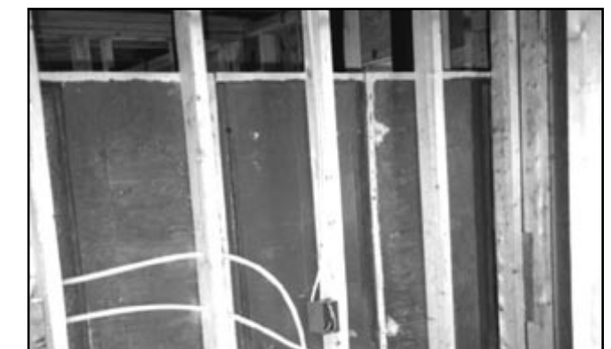
Back of molded shower fixture with whole wall reinforcing installed at factory.
