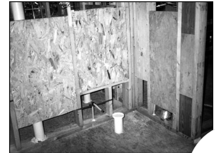
Whole wall reinforcing installed in a Habitat house
