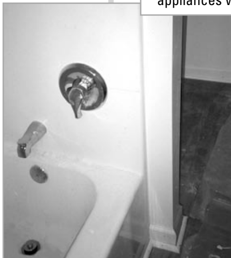
Pressure balanced anti-scald lever control valve in offset location improves usability and safety.
