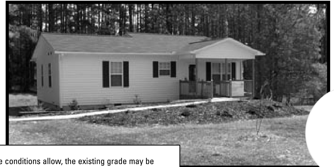
Example of a Habitat house with a gently sloping walk on an earth berm and bridge to provide a stepless entrance.
