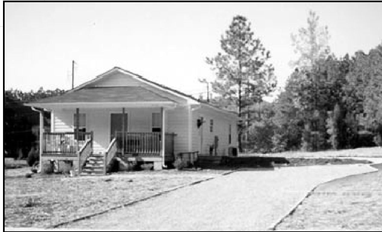
Site placement of this Habitat house took advantage of the existing grade to achieve a gently sloping path on an earth berm at a side entrance.
