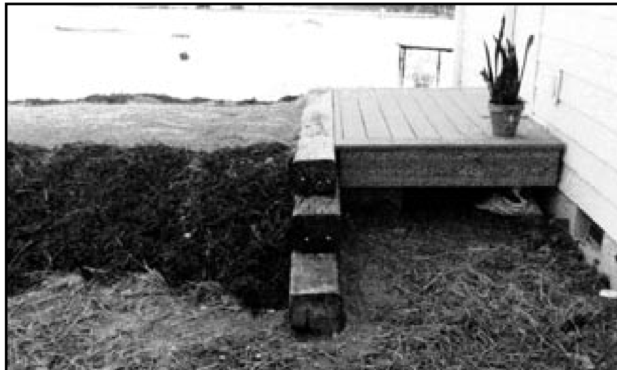
Detail view of the example above where the side stoop has been incorporated as the "bridge" from the retaining wall to house.
